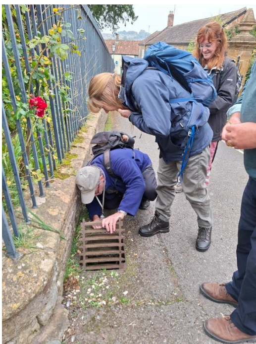
Looking down a drain. Photo © Steve Parker
